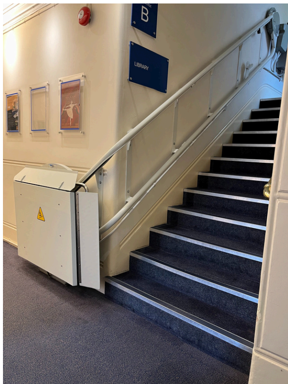
Stairlift platform (250kg weight load) from reception floor to library
