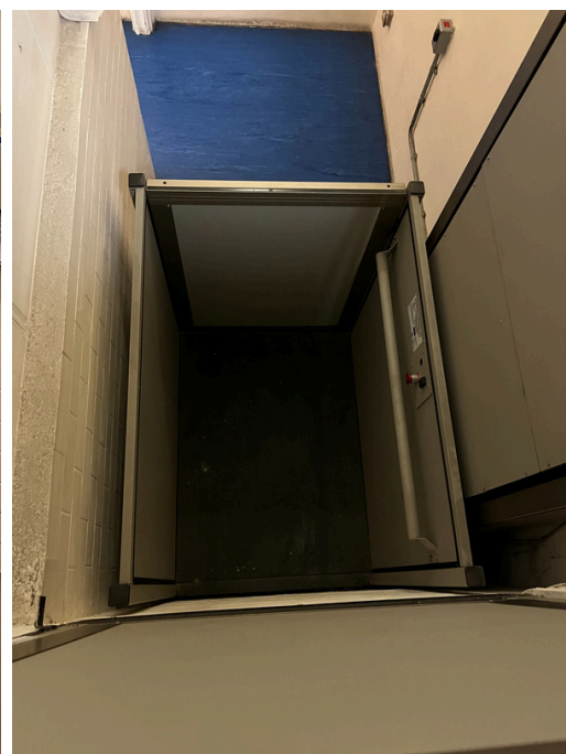
Stairlift platform (340kg weight load) from theatre floor to theatre bar/ foundry/ toilets
